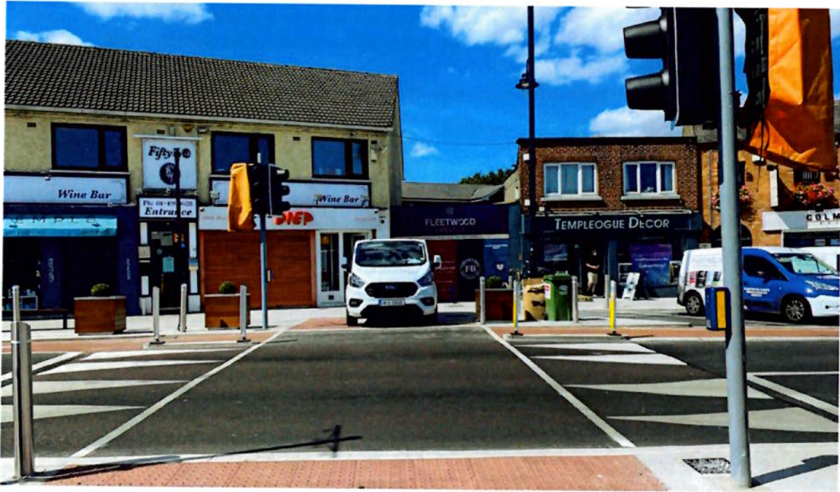
Figure 11 A dedicated on-street loading bay should be provided on the northside of the street
