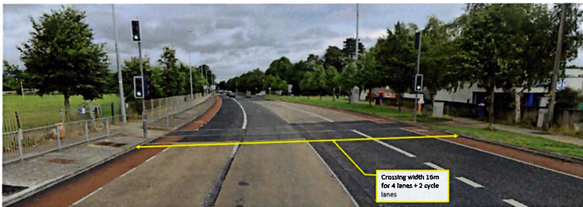
Figure 3 Poor crossing facilities such as this one on the Firhouse Road outside Ballyboden St. Enda's Clubhouse will be replicated by Busconnects
